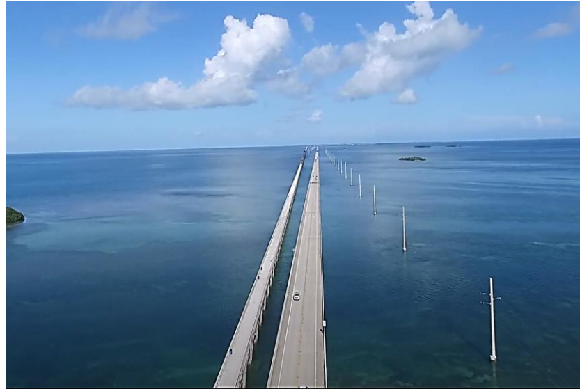
LONG KEY BRIDGE
