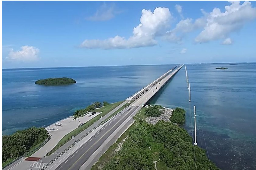
LONG KEY BRIDGE
